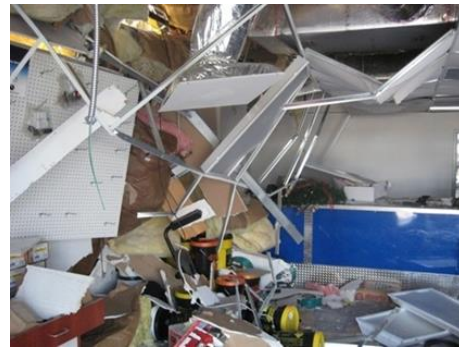
b) Non-Structural Components
