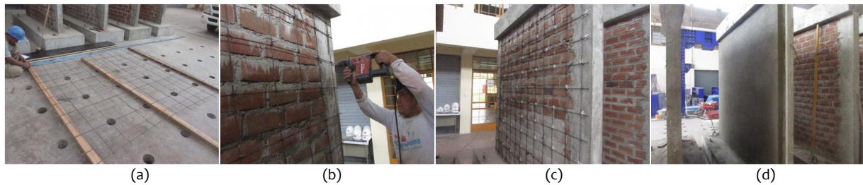
Fig. 12. Retrofitting process on both sides of the masonry wall using steel mesh and cement-sand mortar. (a) Steel mesh fabric. (b) Anchor drilling. (c) Steel mesh anchoring. (d) Mortar coating.
