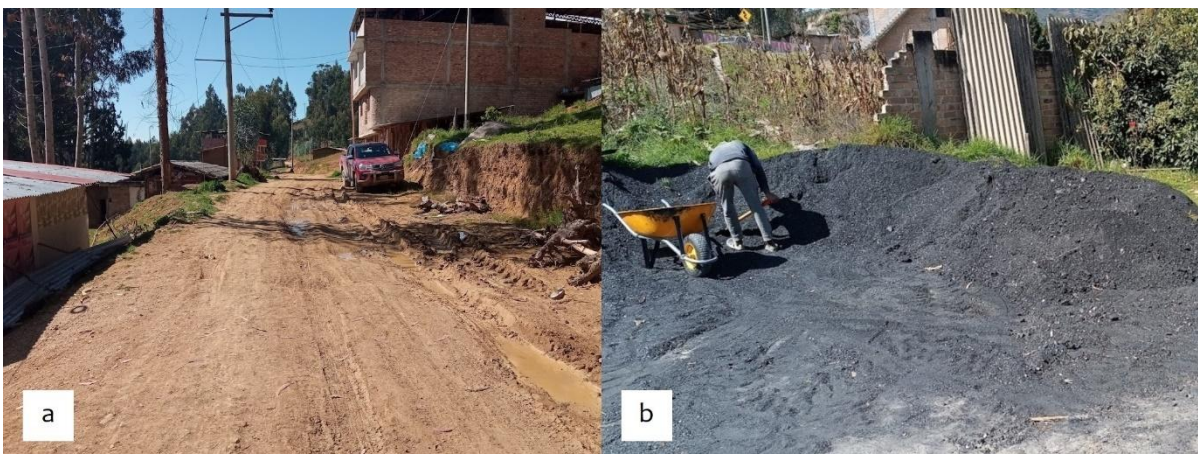
Fig. 2. a) Unpaved road located in Cajamarca, with fine soils at the subgrade level.; b) Mineral coal used in the combustion of artisanal kilns, which generates bottom ash.
